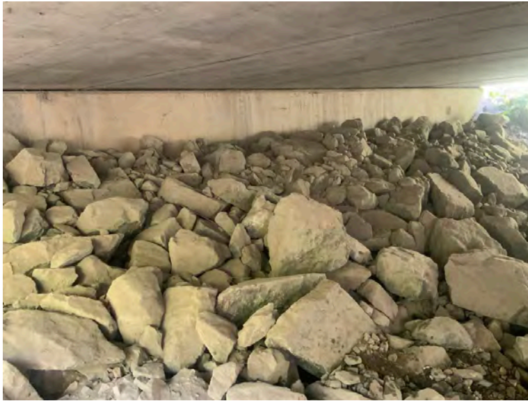
Left Bank Abutment when facing downstream
