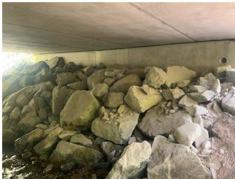
Right Bank Abutment when facing downstream
