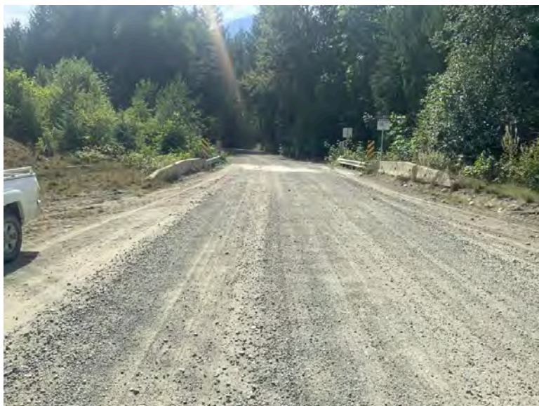
Approach from Right Bank when facing downstream
